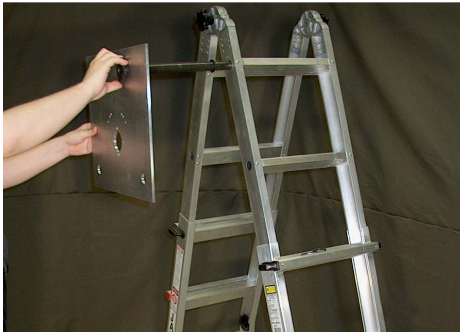
Figure 12: Attach Mounting Plate
